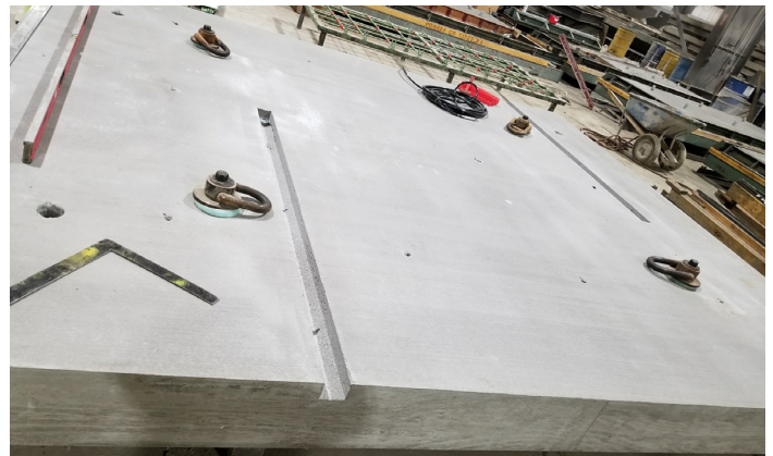
A precast slab being prepared for strip sensor installation
