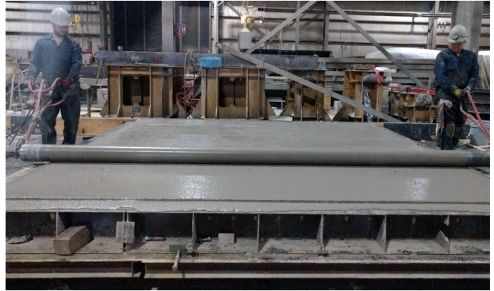
Precast slab surface preparation
