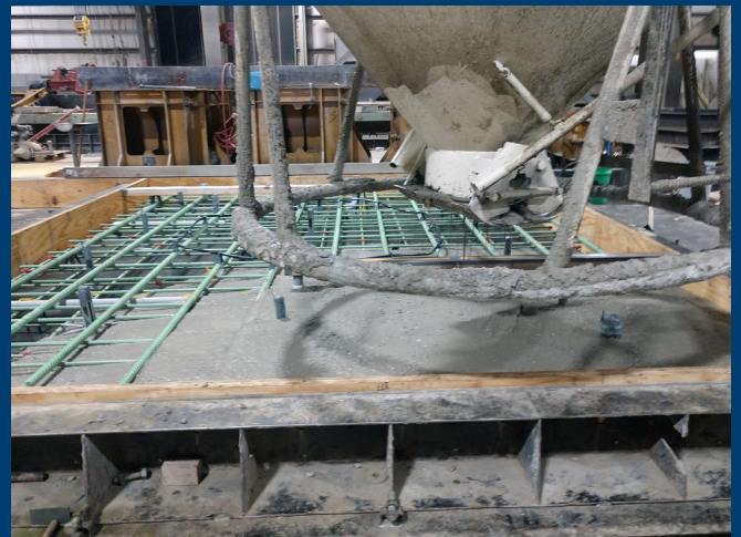
Concrete slabs are manufactured off-site prior to installation
